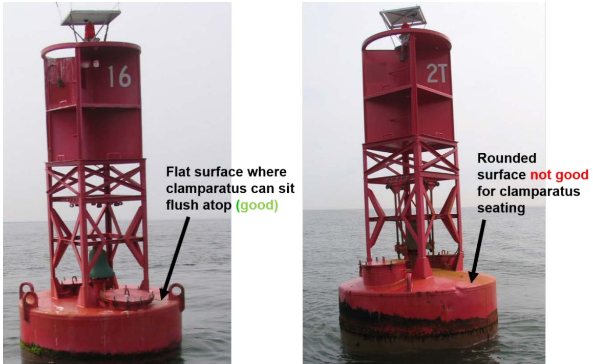
Figure 3: Check top buoy surface during recon to ensure it's flat.
